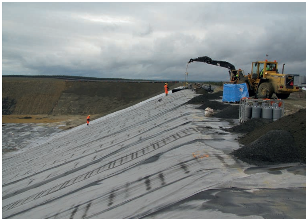
Figure 30. Rubber bitumen used as the covering structure for the upstream slope of the mine dam, Kevitsa Mine. Beneath the bituminous geomembrane liner (+ bentonite liner) is a layer of till with compacted upper layer that borders the blasted rock (left-hand side, see also Figure 29). (Photograph: Timo Regina)
