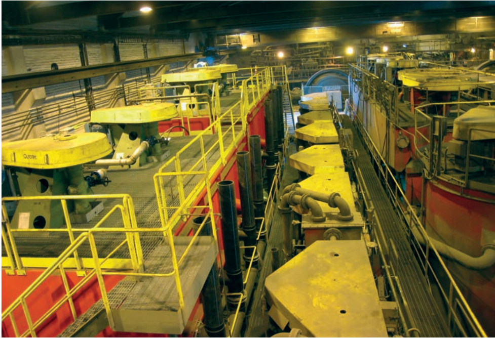
Figure 8. Cu flotation circuit at the Pyhäsalmi mine. (Photo: Pyhäsalmi Mine Oy)
